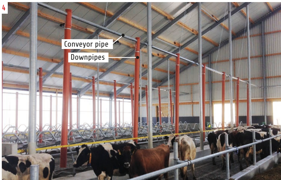
4 Convey- and downpipes inside of the cattle stable
