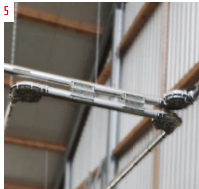
5 Connection of two conveyor lines
