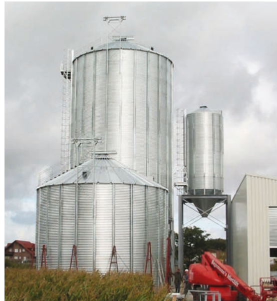
Grain storage with loading silo 75 m 3
