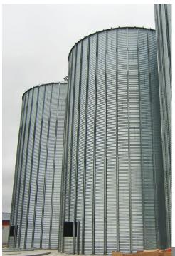
Galvanized flat bottom silo made of corrugated steel profile plates Tailor-made square silo made of steel for optimal use of space
